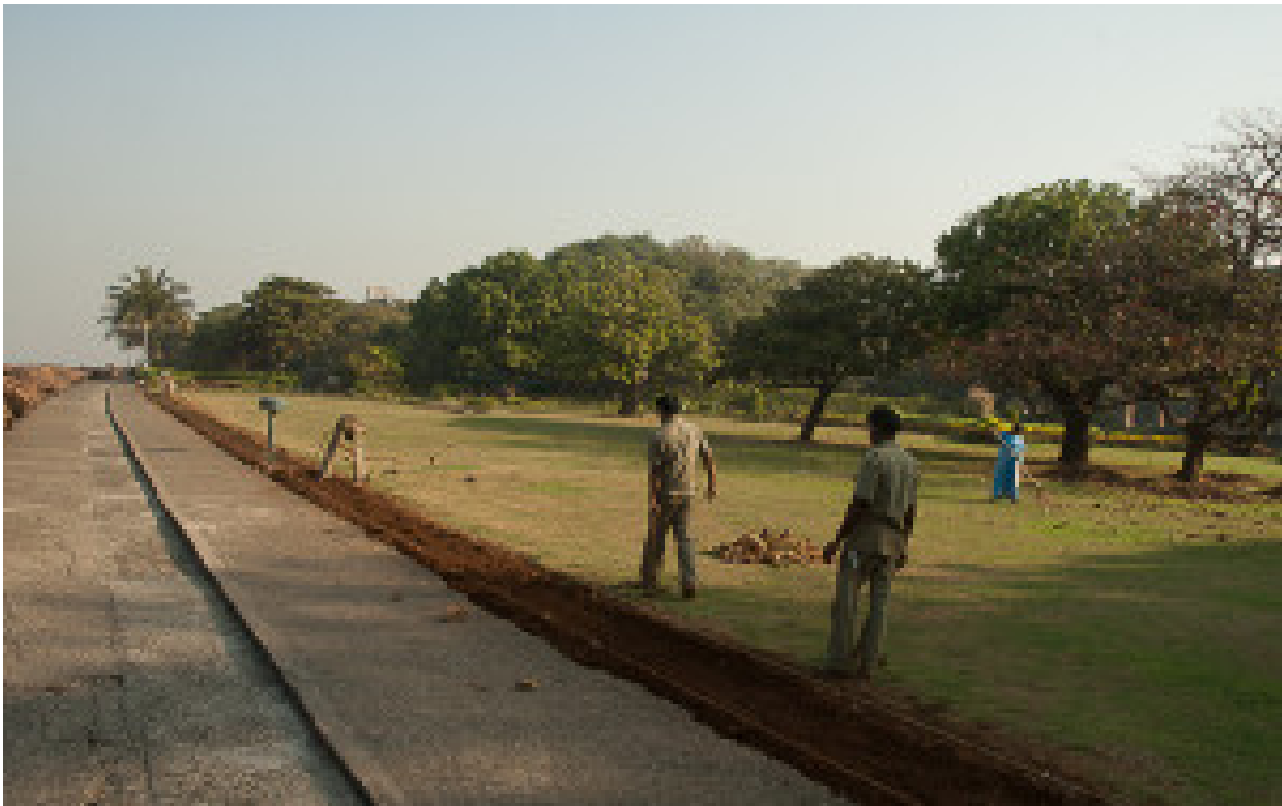
Clearing edge of great lawn for planting.
